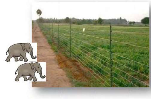
4. Solar Powered High Electric Fences
